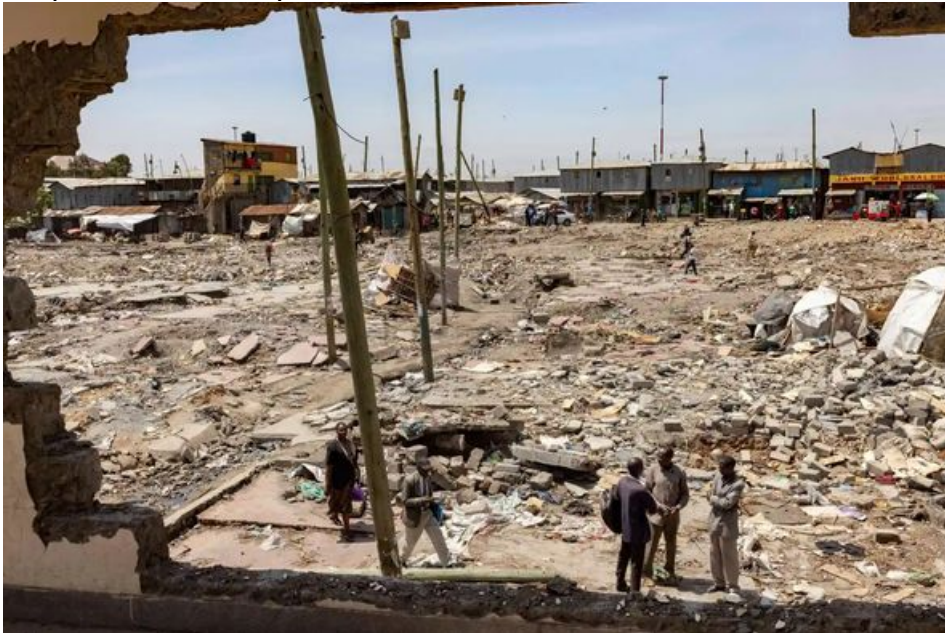
Figure 3-4 Demolition of Mukuru kwa Njenga for the Expressway Source: The Guardian, 2021
