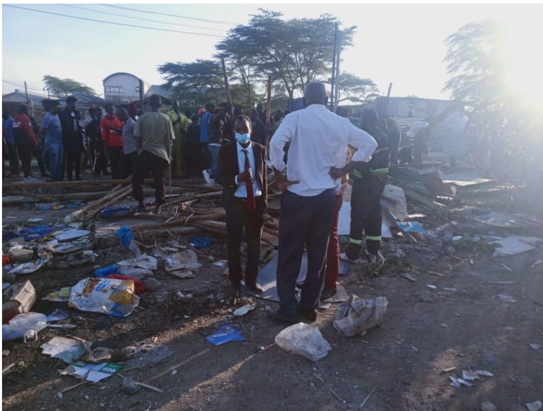
Figure 3-8: Demolitions of Upendo Village in 2021 Source: Taarifa News
