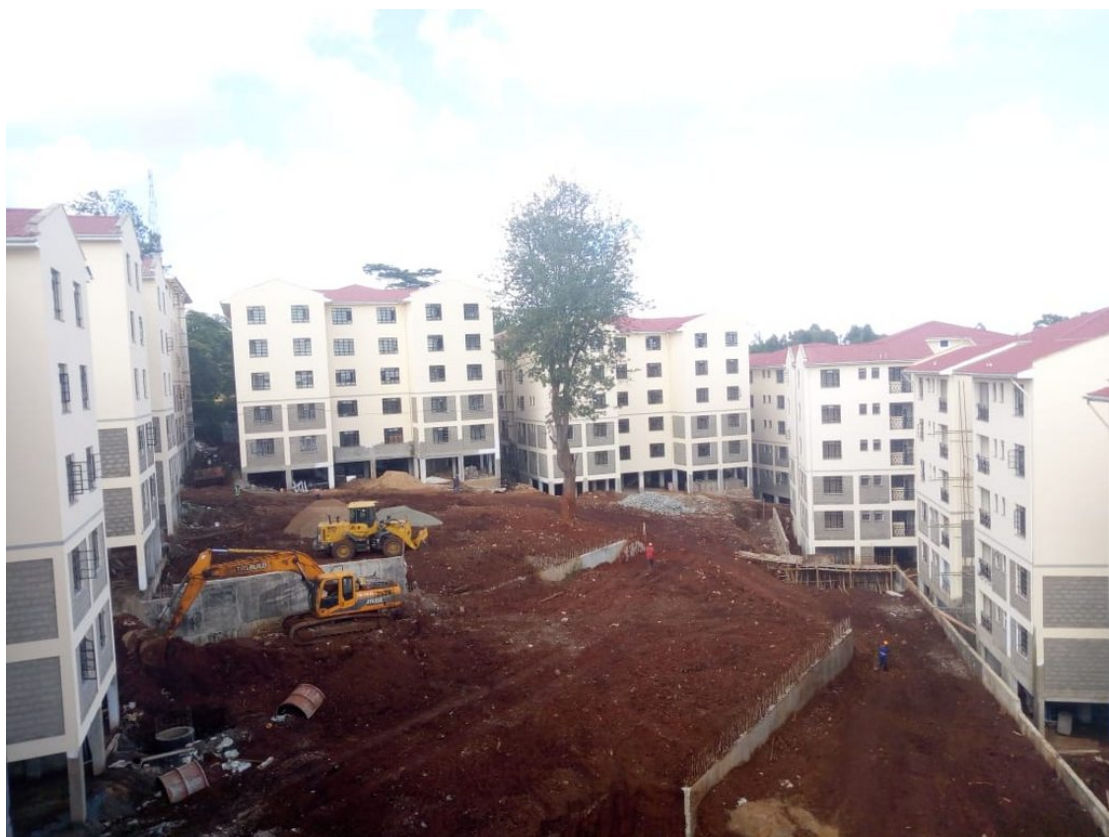
Figure 2-12: Embu Civil Servants Housing Skyscraper city (2022) 17
