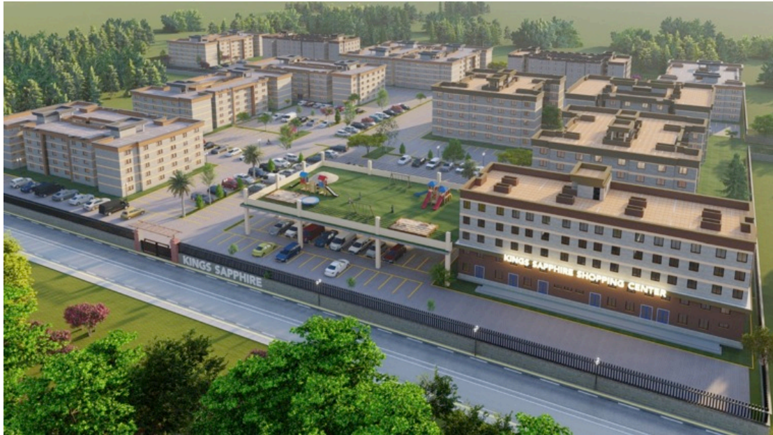
Figure 2-6: Kings Sapphire project, Nakuru Source: Government of Kenya, 2022
