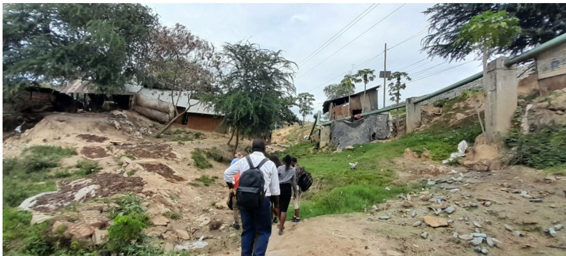
Figure 4-12: Demolished area for road construction in Mkupe Changamwe Source: Author
