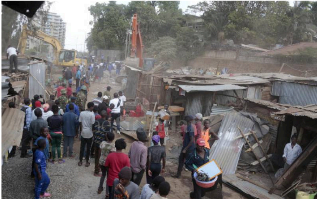
Figure 3-7 Demolition of Deep Sea, 2021 Source: Imam, Masoud (2021) The Standard Newspapers 21
