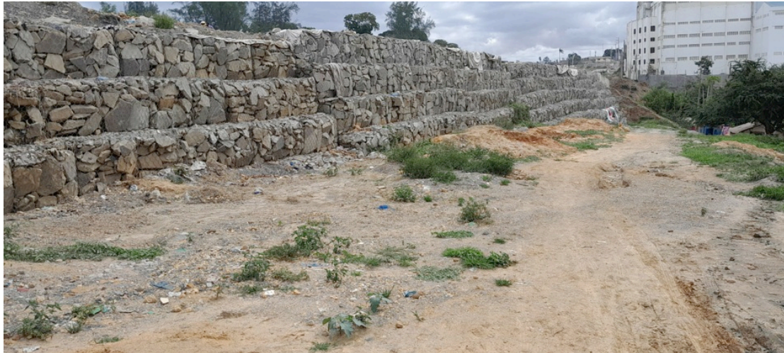
Figure 4-11 Cleared area for road reserve in Mkupe, Changamwe Source: Author
