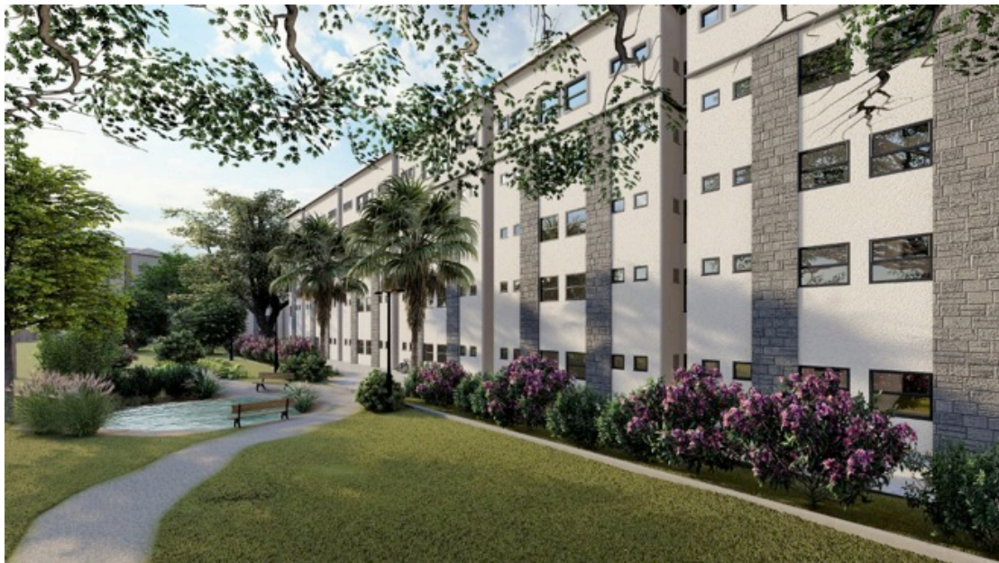
Figure 2-7: Kitui County Affordable Housing Project Source: Government of Kenya, 2022
