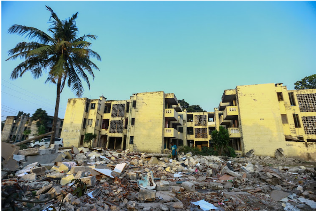
Figure 4-5: Demolition of Buxton Estate in March 2021 Source: John Chesoli
